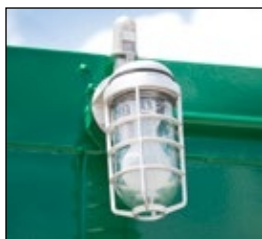
Vapor-resistant exterior light with photocell
